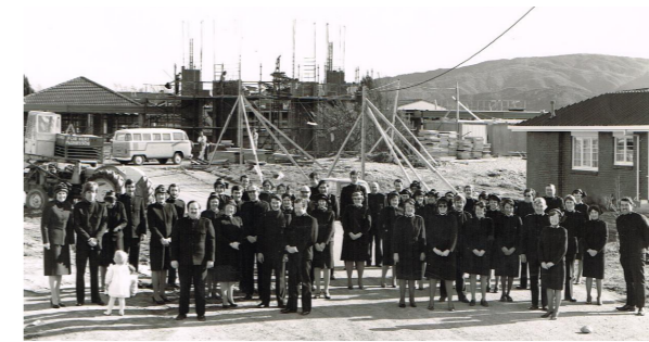
Booth College of Mission building under construction - 1983.
