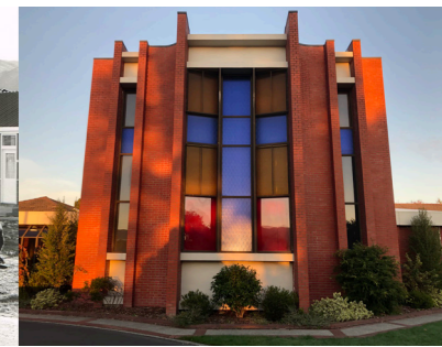
Facade of the Booth College of Mission - 2019.
